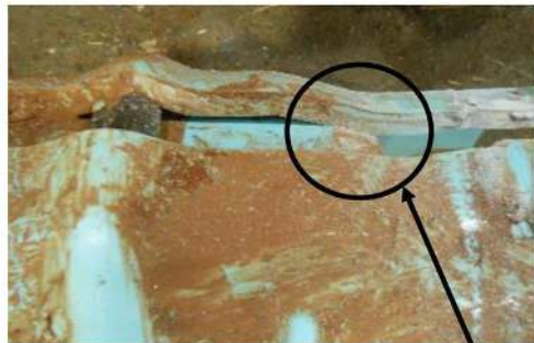
Overstabbing wedged against the inside of the bell
