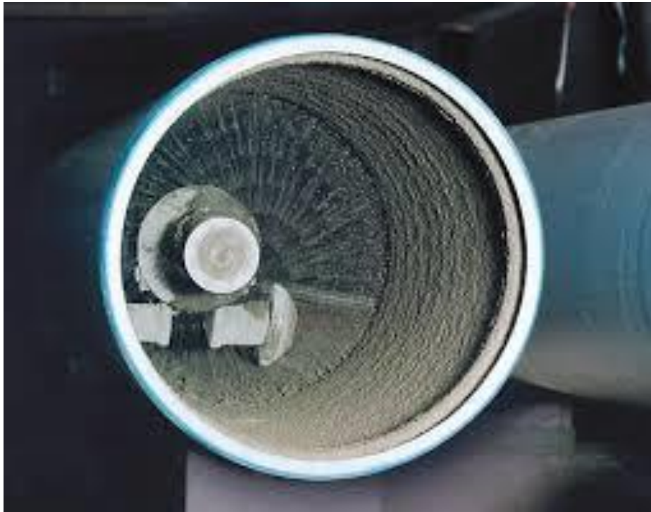
Cement Mortar Lining
